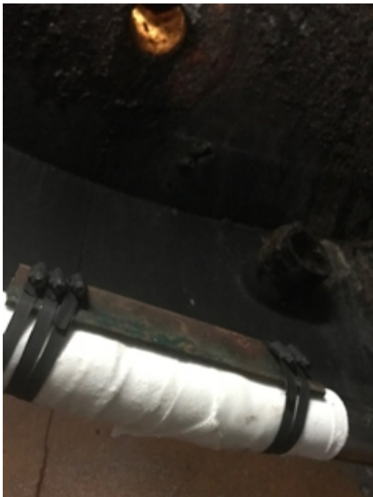
The completed repair with steel deflector plate tied to the top for added protection from future debris
