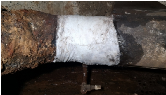
Repair to the section of pipe with the welded joint
