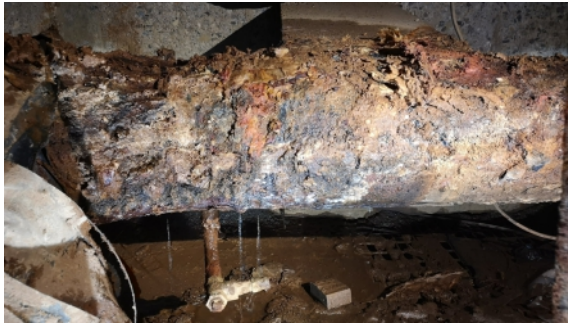
Section one of the pipe required a challenging repair around a welded joint
