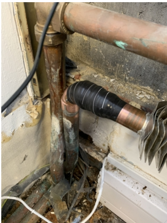
Completed repair with Wrap & Seal tightly applied over the leak area, sealing the joint
