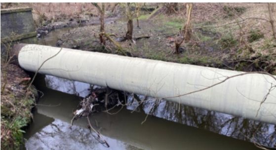
Pipe bridge wrapped along 20m length with SylWrap
