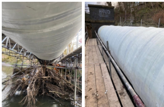
Completed repair, seen from underneath pipe bridge and from the scaffold constructed for application
