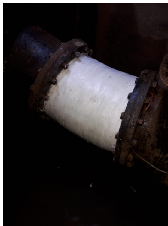
Completed repair showing SylWrap HD wrapped around a 22 degree elbow joint on a 450mm main
