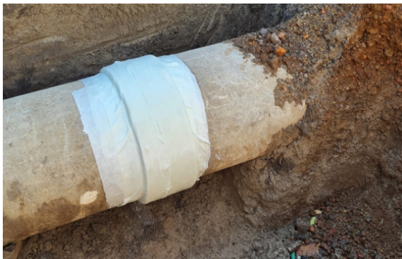
SylWrap HD encompassed the sleeve, completing the repair
