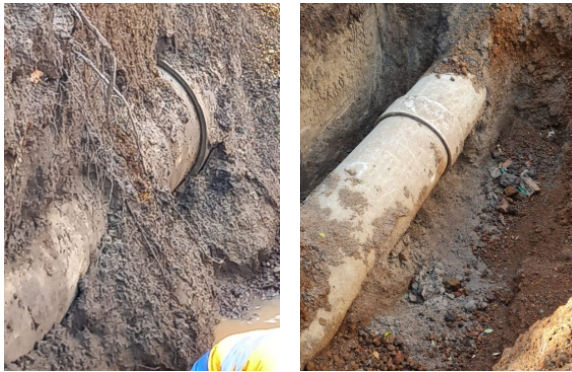
A trench was dug to attend to the buried pipeline
