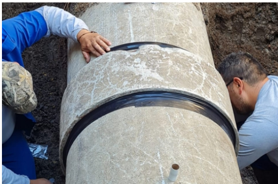
Wrap & Seal was used to reinforce Superfast Copper
