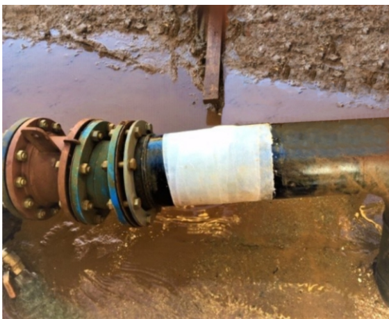
The completed repair reinforced with a SYL633HD SylWrap Pipe Repair Bandage
