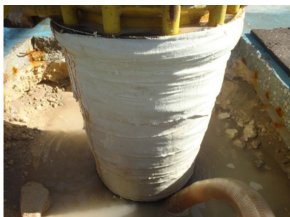
The floor was excavated to access an underground section of the stub with the whole pipe encompassed in a protective sleeve of SylWrap HD
