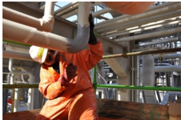
Industrial Metal was applied via a hand tool by an engineer to encompass the entire elbow
