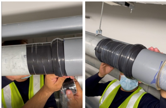
Once the ridge reached level height with the step, wrapping continued to encompass the joint
