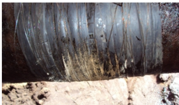
Multiple Wrap & Seals sealed the crack on the line
