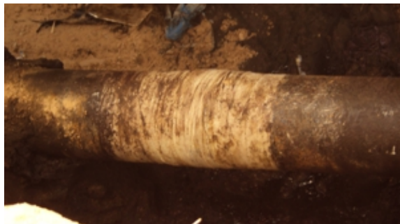
SylWrap HD reinforced and protected the repair
