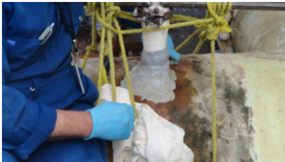
A PTFE plug was fixed in place using Sylmasta AB
