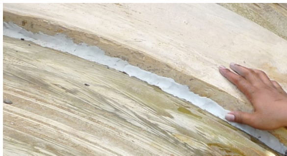
AB Original pushed into seal all gaps in the pipe
