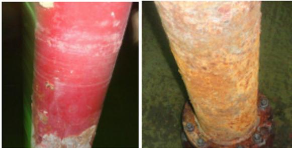
Lower sections of the pipe were badly corroded
