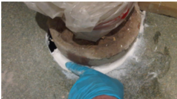
The putty was smoothed off using a little water and a filling knife as the application continued
