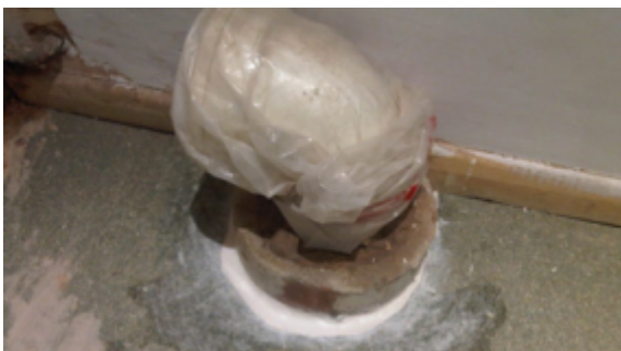
The completed repair with all gapping sealed and the waste pipe successfully plumbed in
