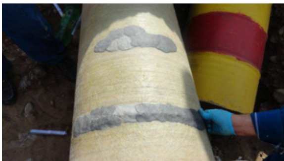
The putty cured to form a material hard as steel over the weakened areas
