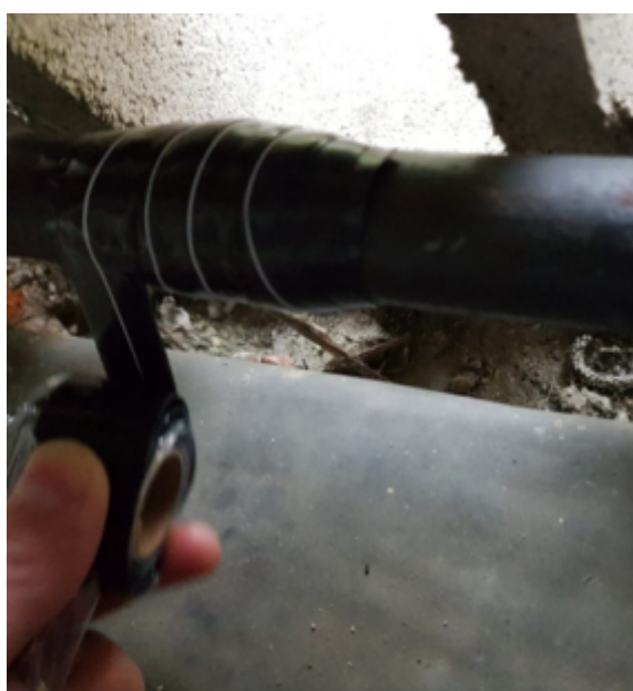
The tape was then pulled under the pipe and up through the 30mm gap between the pipe and the back wall
