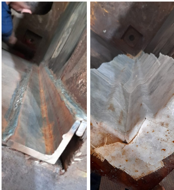
New metal corners were welded to reinforce all four corners of the chromic acid tank. These corners were then encompassed with SylWrap HD
