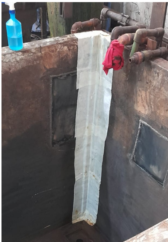
Patches of SylWrap pressed and smoothed over each corner created a watertight seal between the weld and the existing iron frame of the tank
