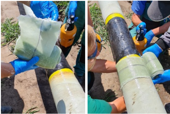
SylShield was activated with water and then wrapped over heat shrink sleeves covering the welded joints
