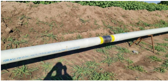
Sections of pipe were welded together (black area) to fabricate the line above ground prior to HDD
