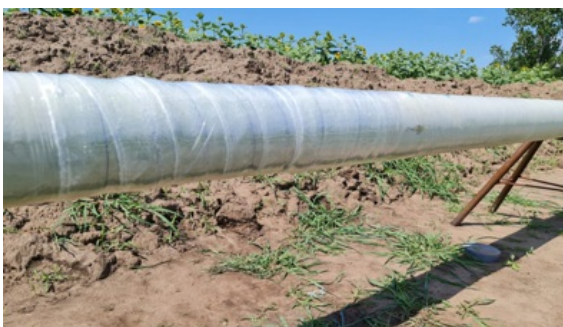
Once the line had been protected, it was ready to be pulled through the ground and installed via HDD
