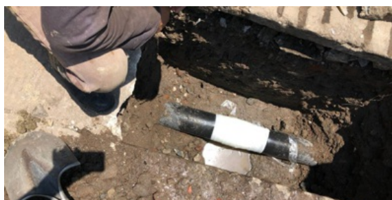
After the leak was sealed with Wrap & Seal, SylWrap HD provided an effective replacement for the coating
