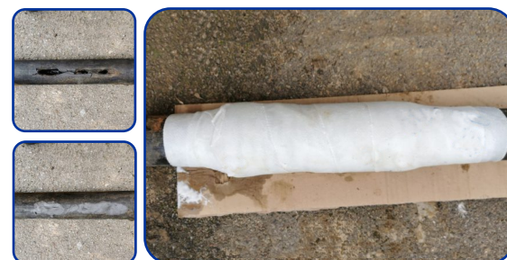
When pressure can be stopped, epoxy putty fills in holes, cracks and missing sections
