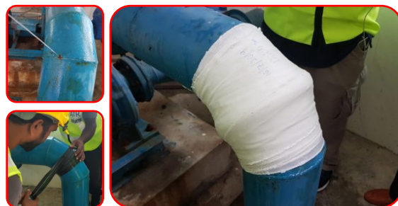
When pressure cannot be stopped, pipe burst tape is wrapped tightly around the leak area
