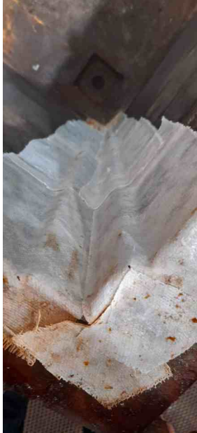
New metal corners were welded to reinforce all four corners of the chromic acid tank. These corners were then encompassed with SylWrap Bandage
