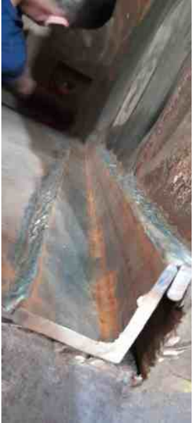
New metal corners were welded to reinforce all four corners of the chromic acid tank. These corners were then encompassed with SylWrap Bandage
