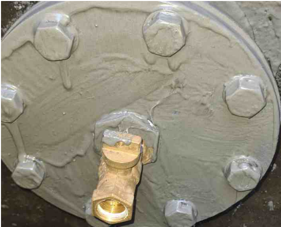
Liquid Metal shielded the flange plate from corrosion
