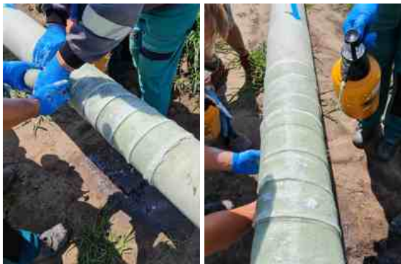
After being smoothed, SylShield cured to form an ultra hard shell protecting the steel pipe
