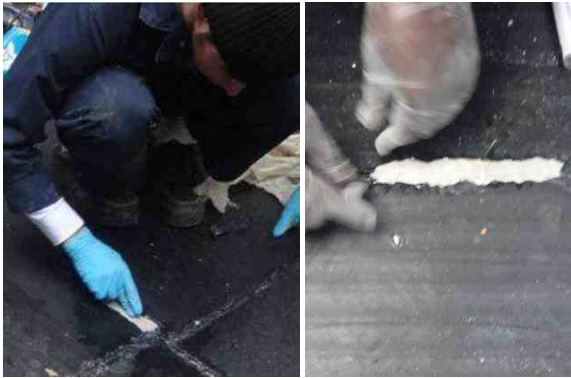
AB Original was pushed into each gap before being smoothed off with water and a hand tool
