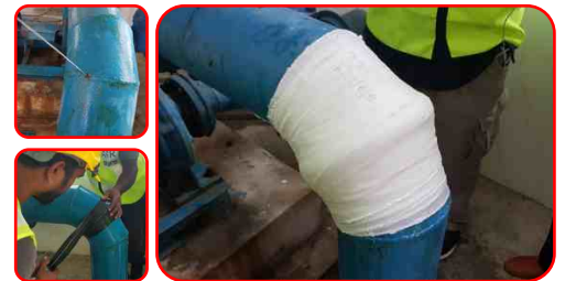
When pressure cannot be stopped, pipe burst tape is wrapped tightly around the leak area
