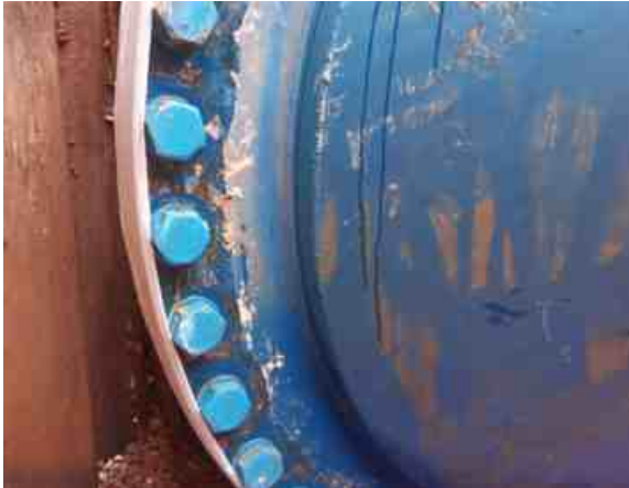
The flange connected a steel pipe to a chlorine tank
