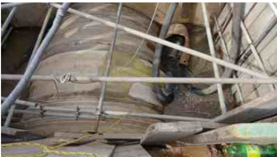
The line successfully sealed prior to being re-buried
