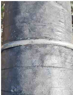
SylWrap CR was carefully applied to the whole line, providing further reinforcement and protection
