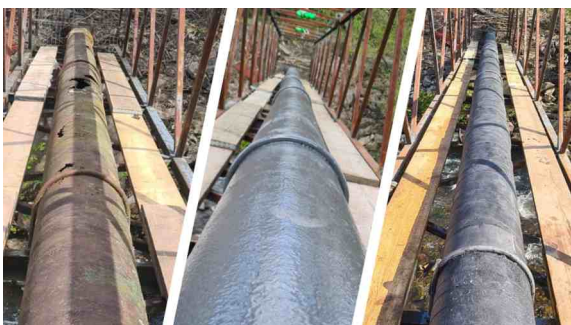
SylWrap CR was carefully applied to the whole line, providing further reinforcement and protection
