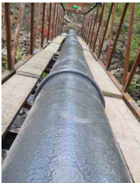
Liquid Metal was painted onto the pipe, curing to form a new, impermeable metallic outer surface
