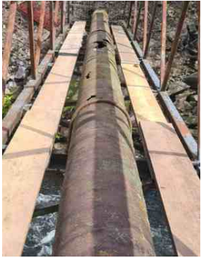
Corrosion had breached the pipe in several places
