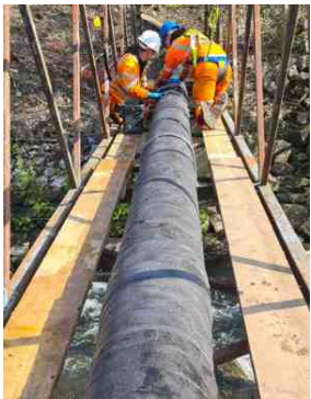
SylWrap CR was carefully applied to the whole line, providing further reinforcement and protection
