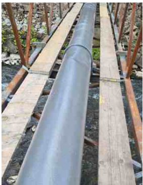
Liquid Metal was painted onto the pipe, curing to form a new, impermeable metallic outer surface
