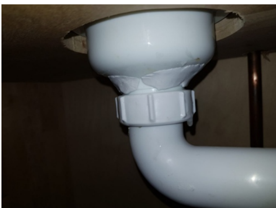
The putty hardened, permanently sealing the cracks in the pipe and preventing any more water from escaping when the sink drained
