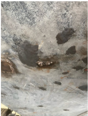
AB Original Black Epoxy Putty filled in all holes
