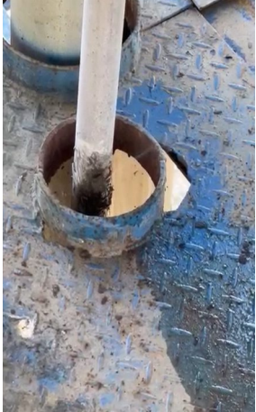
Alcohol juice was spraying through a pinhole leak at a pointed where the line passed through a circular hole in the upper floor of a platform
