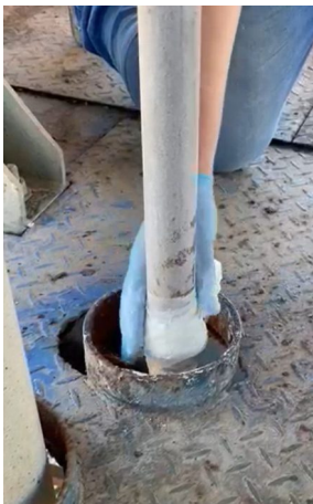
The repair was reinforced and protected with SylWrap HD Pipe Repair Bandage
