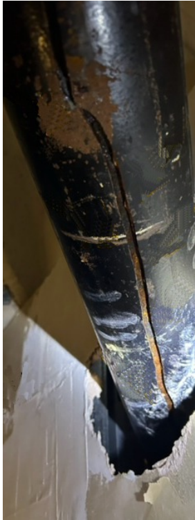
Water escaping through the 1.05-metre long crack in the downpipe had saturated surrounding plasterboard and was now leaking into a nearby hospital ward
