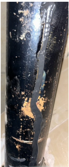
The crack was sealed by extruding CrackSeal directly into it. The entire length of pipe was then reinforced with SylWrap for a permanent repair
