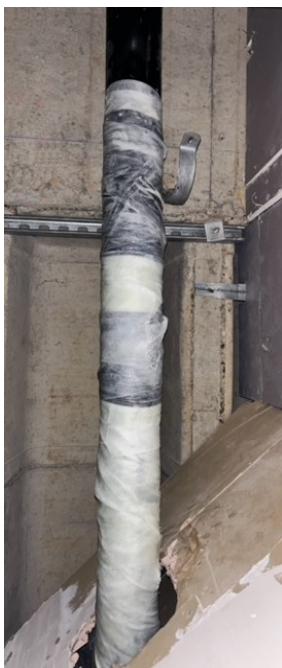
The crack was sealed by extruding CrackSeal directly into it. The entire length of pipe was then reinforced with SylWrap for a permanent repair
