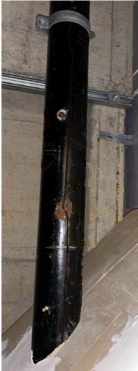
Water escaping through the 1.05-metre long crack in the downpipe had saturated surrounding plasterboard and was now leaking into a nearby hospital ward
