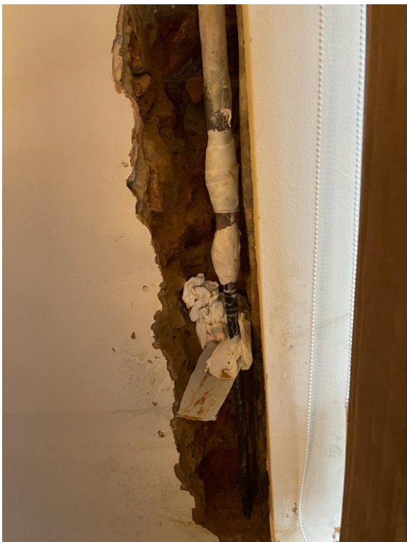
Despite the space constraints in the wall, the pipe was repaired using Wrap & Seal and SylWrap HD
